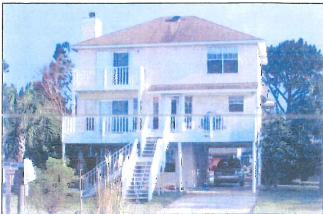
Elevated home on pile foundation
